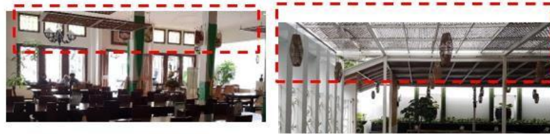
Figure 3 The Ceiling in Paviliun Sunda Source: Author's documentation, 2018
