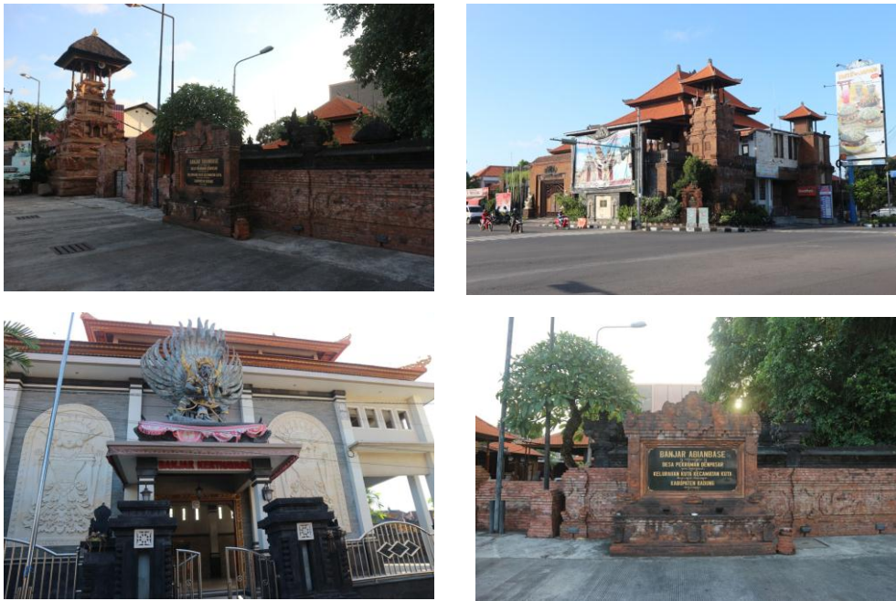
Figure 1. Some surveyed buildings of bale banjars Source: Mahastuti and Utami, 2020.
